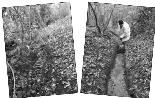
Drainage ditches before and after work in 2012
