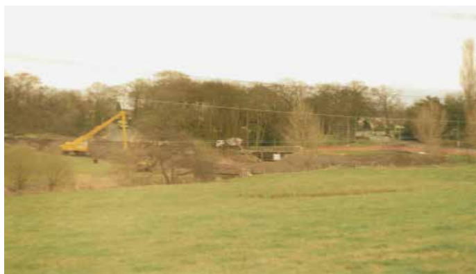
Work in progress, view towards Valley Road.
