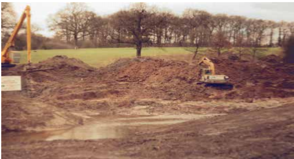
Landscaping in progress. The sign tells that a 'New Amenity Lake' is being constructed, this is now the pond near to Church Lane.
